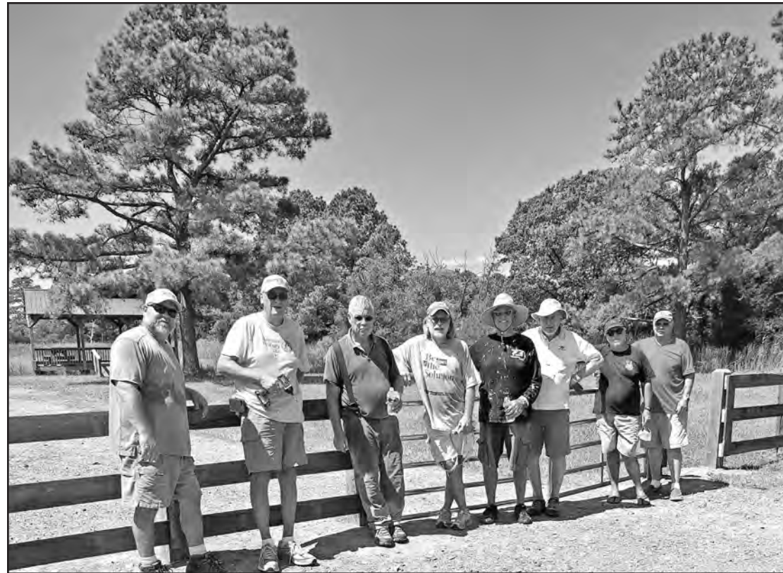
The Mathews Rotary Club's annual community service project this year was construction of a fence to protect Bayside in Bavyon from vandals. The property is owned by the Mathews Land Conservancy and is a popular stop on the Tour de Chesapeake. Among those working on the project were, from left, Andy Eubank, Ron Lambert, Jack White, Brian Russell, Karl Braun, Dick Hellier, Stan Allen and Chuck Dawson.
